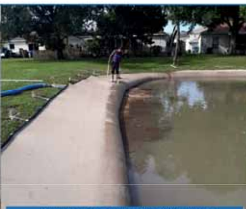
DURING: INSTALLING SOX EROSION CONTROL
